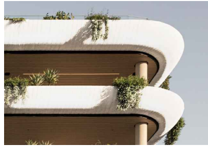
balconies and bands with painted render finish (cr)
