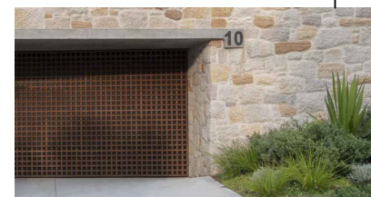
stone front fence (st) garage gate
